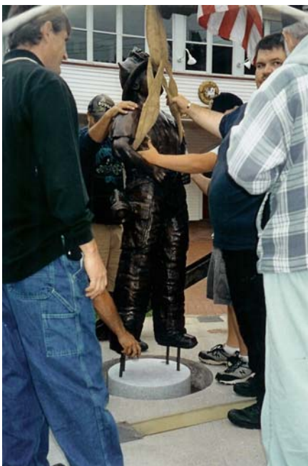
Steel rods were threaded into the feet of the bronze figures while D&C reporter Victoria Freile records her visit for the Rochester based newspaper.
