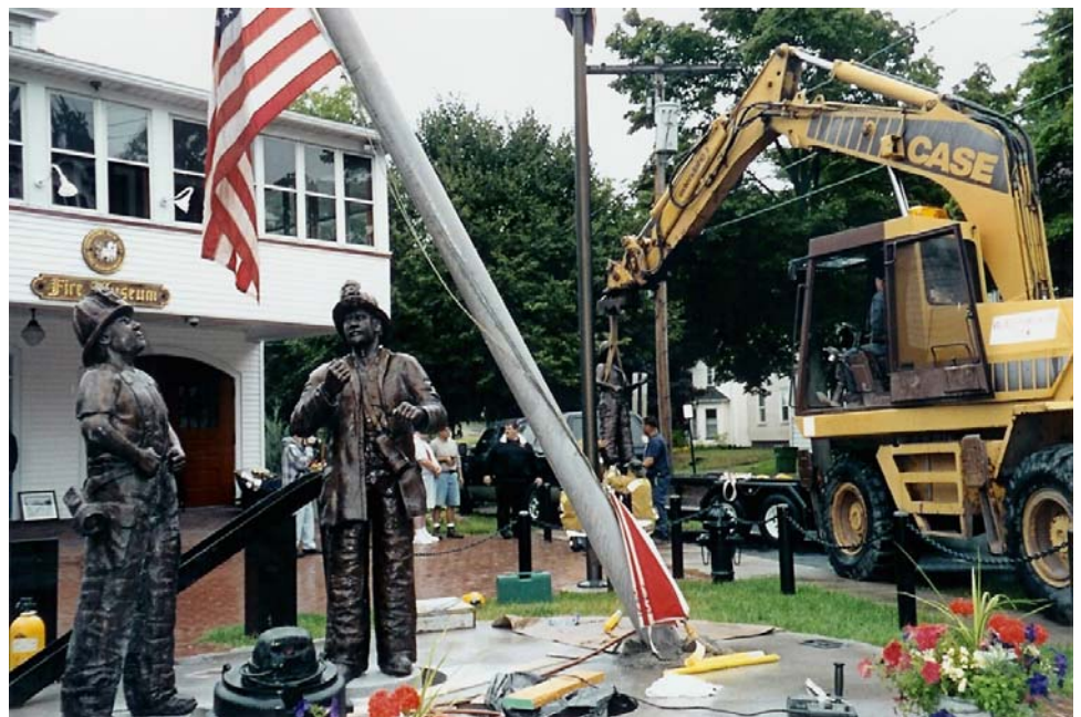
Steel rods were threaded into the feet of the bronze figures while D&C reporter Victoria Freile records her visit for the Rochester based newspaper.
