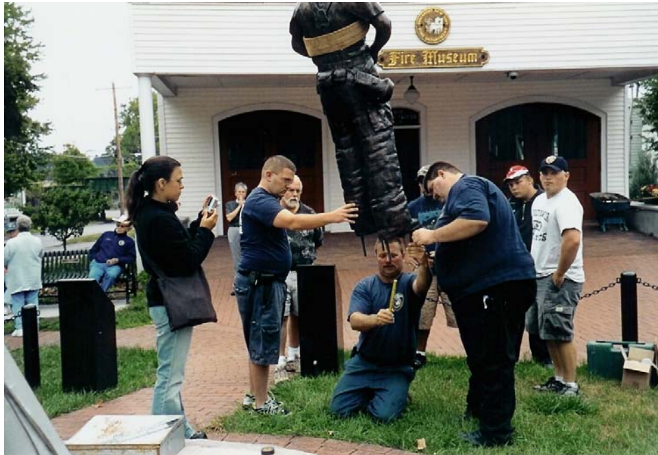
Steel rods were threaded into the feet of the bronze figures while D&C reporter Victoria Freile records her visit for the Rochester based newspaper.
